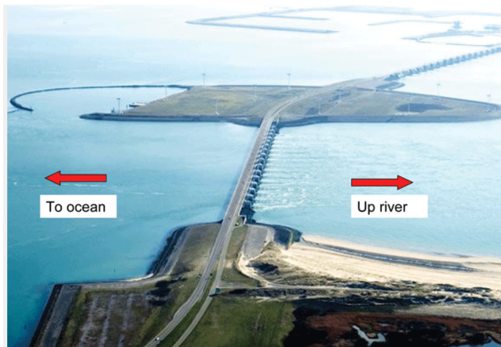
An image from Malcolm Bowman's presentation on storm surge barriers, showing a view of a segment of the Delta Project, in the Netherlands. The system is composed of a mixture of elevated natural sand dunes, tidal gates (normally open), elevated highways and shipping gates. The photo was taken during flooding (incoming) tides. During storm surges, gates are lowered from the highway for protection.
