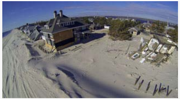
Damage to homes along the beach in Mantoloking, New Jersey, left by Hurricane Sandy five months after the storm. Taken from a miniature Quadcopter along the coast of Mantoloking. (Photo by Wendell A. Davis Jr./FEMA)
