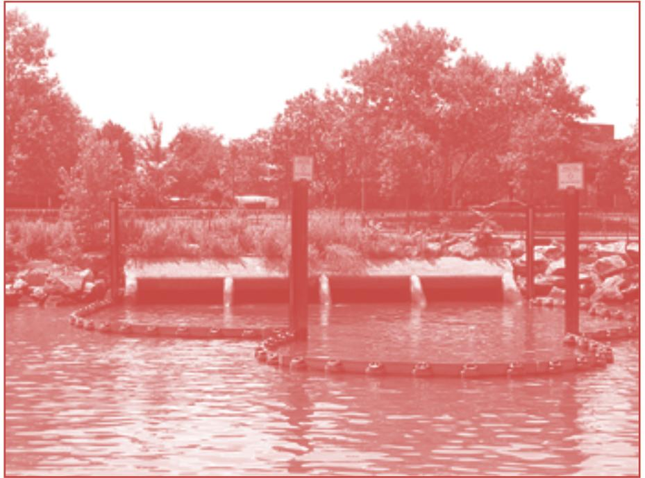
A boom, or floating barrier, captures floatables discharged from a combined sewer. NYCDEP skimmer vessels remove floatable debris from boomed CSO outfalls. Photo courtesy of Dennis Scannell, Hydroqual, Inc.
