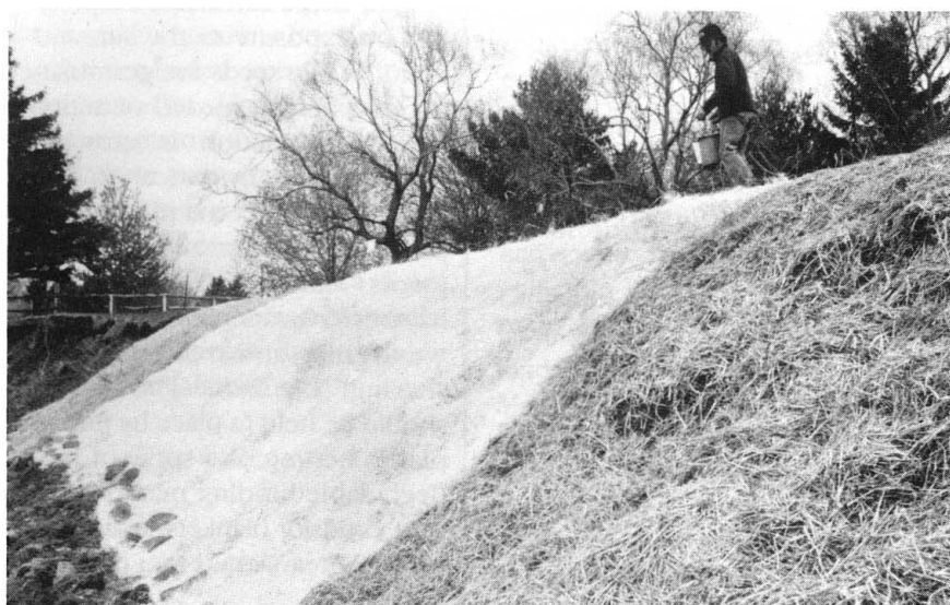
Figure 23. Straw, held in place by jute and plastic netting (left), and excelsior blanket mulch (right) were critical in protecting the seed, transplants, and soil against the elements.
