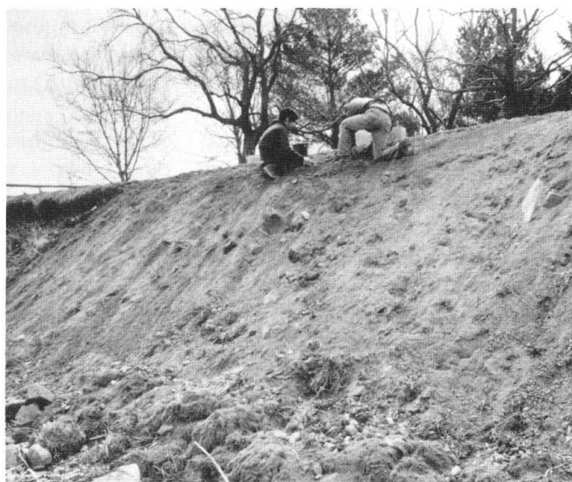
Figure 22. The B. Forman Park Demonstration Project involved smoothing a steep, moderately eroding coastal bluff to a gentler slope and planting that slope with a variety of deep-rooted conservation vegetation.
