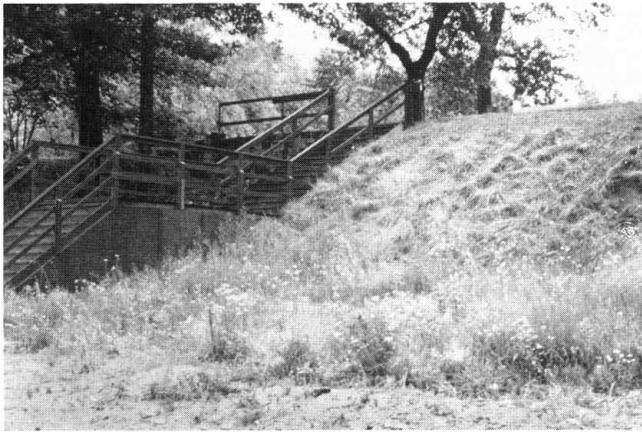
Figure 11. Pedestrian traffic on bluffs can destroy the natural vegetation, allowing the formation of gullies. Instead of surface pathways, wooden stairs should be constructed for access up and down the bluff.
