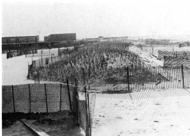
Figure 17. The “new” dunes were fenced to reduce the amount of foot traffic and planted with beachgrass.
