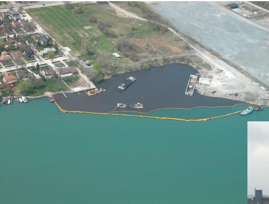
REMEDIAL DREDGING APPLICATION
