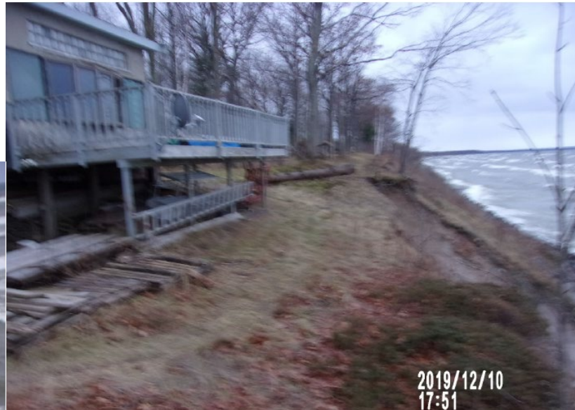
Looking to the South
