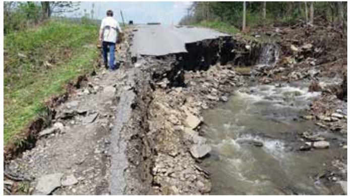
*East Valley Road, north of Branchport, NY. Floodwaters were beyond the capacity of existing ditches and culverts. Many area roads were damaged from the velocity and volume of the floodwater. Photo: Courtesy of Dave Enty (NWS Binghamton).*
