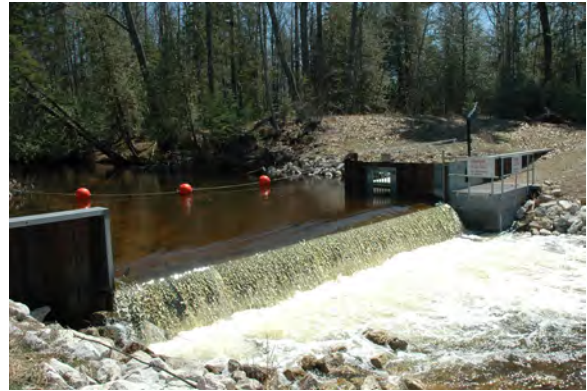
Example of a low head barrier. Photo: M. Siefkes, Great Lakes Fisheries Commission
