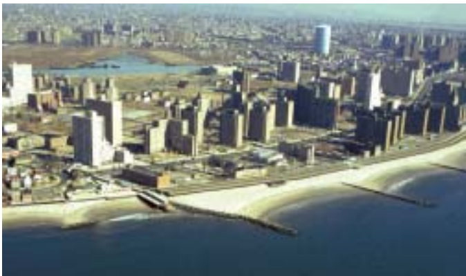
Erosion control structures and beach nourishment have helped slow down erosion and preserve the beach in front of the heavily-developed Coney Island shoreline. Photo courtesy of Jay Tanski
