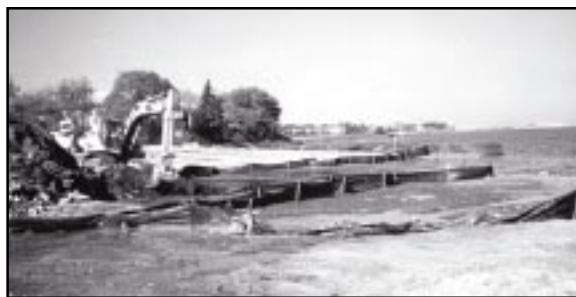
Excavating the site.
