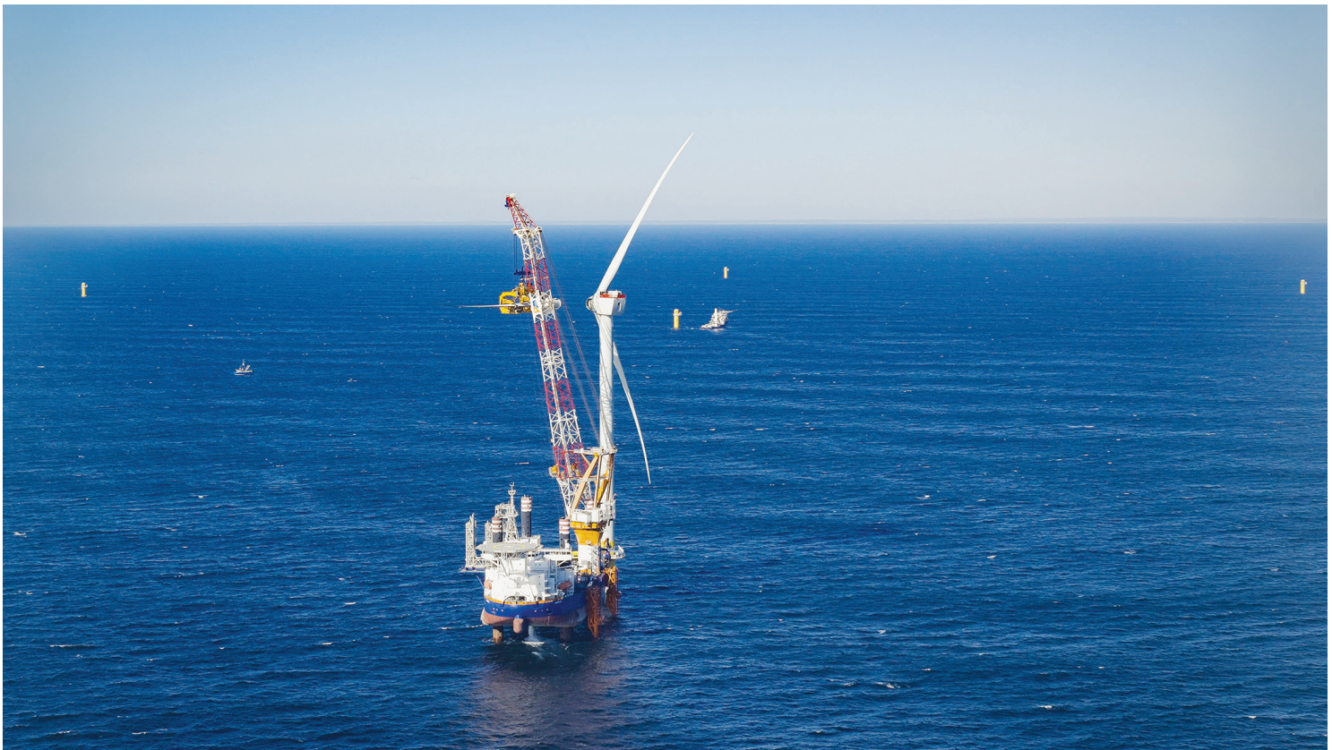
Construction of the first offshore wind turbines off Montauk, Long Island. South Fork Wind , by Orsted and Eversource, generates approximately 130 MW to power approximately 70,000 Long Island homes. Source: Orsted .
