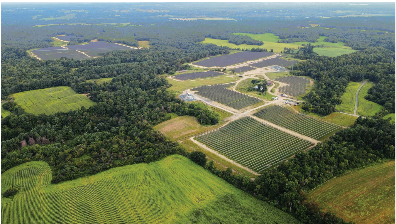
CS Energy is one solar company that partners with NY State to build industrial solar arrays. Completed in 2021, this 27 MW solar array has enough electric capacity to power more than 4,934.
