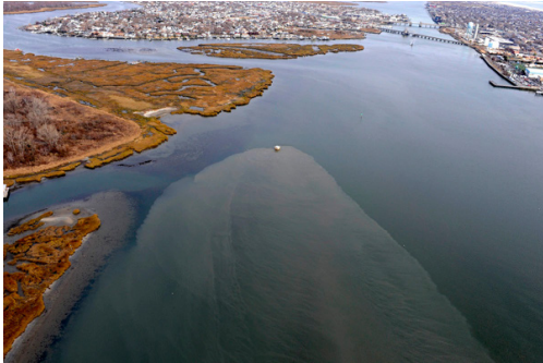
Storm surge from Hurricane Sandy caused significant damage to the Bay Park Sewage Treatment Plant in East Rockaway, NY, which treats 50-85 million gallons day of waste water from 40 percent of Nassau County residents. Credit: Doug Kuntz/Newsday
