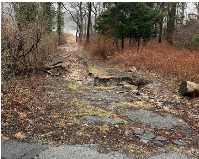
Erosion caused by stormwater runoff in the Hitherbrook Road area. Credit: Village of Head of the Harbor.
