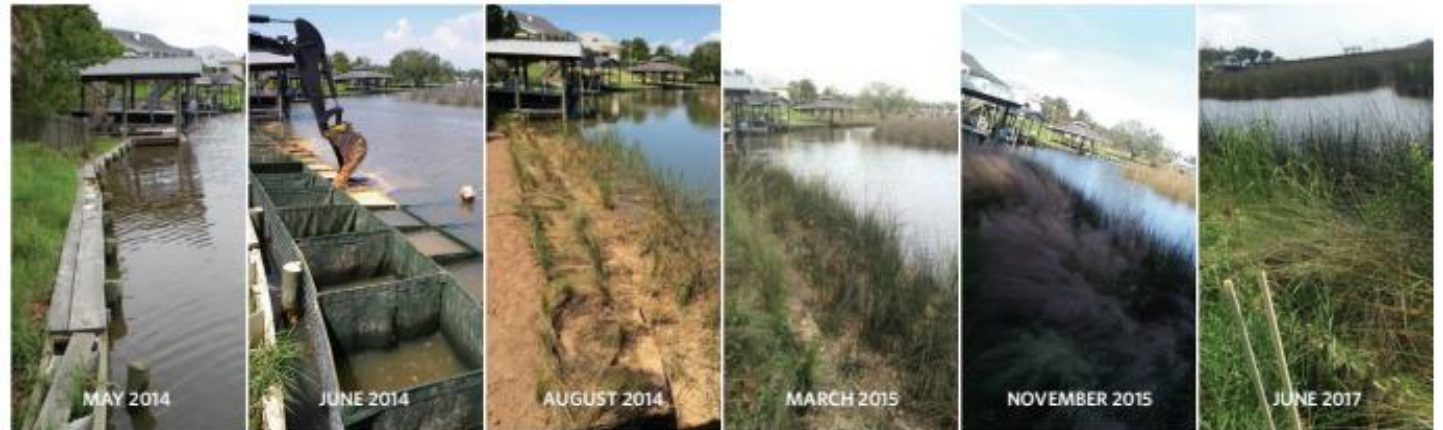
Living shoreline retrofit of a bulkhead seawall in Mobile Bay, Alabama (The Nature Conservancy)
