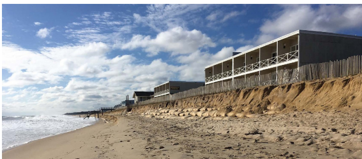
Exposed sand bags due to beach erosion. Credit: Kathleen Fallon
