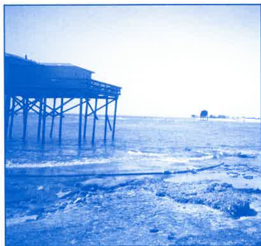
Breach at Westhampton.
