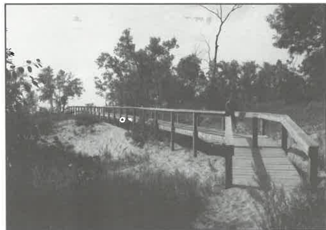
The wooden dune walkover is designed to protect the sand dune from heavy foot traffic.
