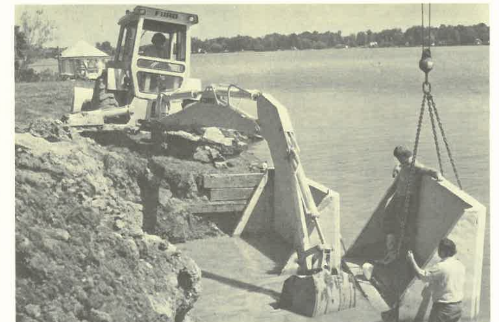
Two methods of erosion control: a do-it-yourself project building gabions; and a construction project using concrete bulkheads. Both measures can save your money now and your shoreline property next year.
