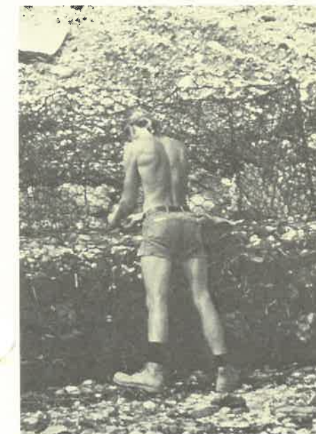
Two methods of erosion control: a do-it-yourself project building gabions; and a construction project using concrete bulkheads. Both measures can save your money now and your shoreline property next year.
