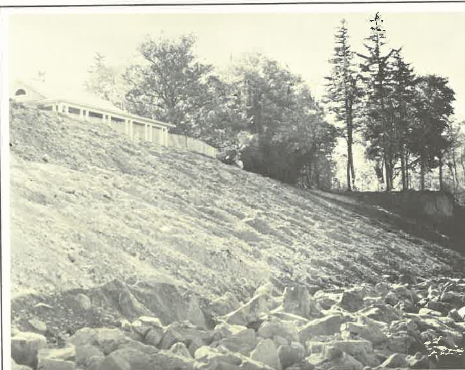
With the toe of this Lake Ontario bluff now protected by a rock revetment, the slope has been regraded in preparation for vegetative ground cover, which can help stop erosion.
