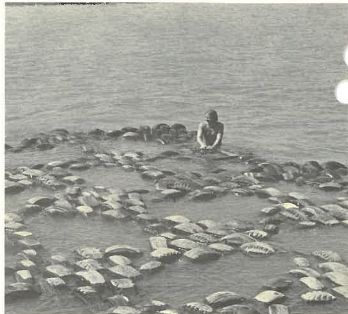
Regional Marine Specialist, Rob Patten (shown above) was one of the many Dunkirk residents who helped to build the scrap tire breakwater.
