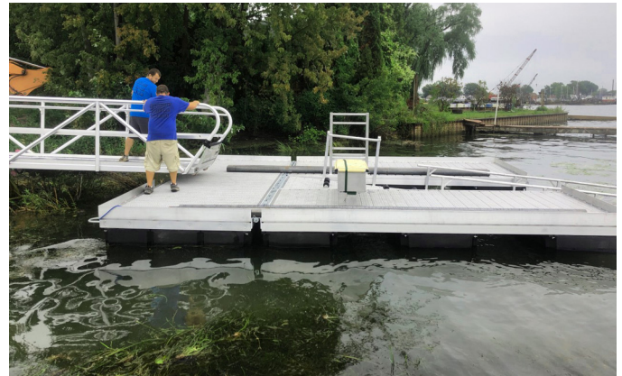
A NY Great Lakes Basin Small Grant funded the installation of this ADA-compliant kayak launch ramp along Lake Ontario. Photo: Maxine Appleby, Wayne County SWCD
