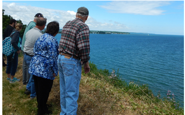
NYSG shoreline tour participants view a bluff protection and stabilization project along Lake Ontario. Photo: H. Weitzner
