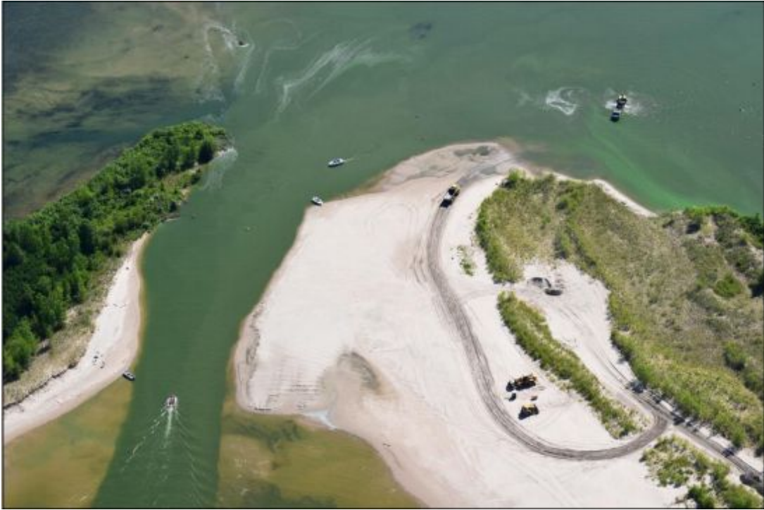
Figure 19: 2016 Inlet dredging operation
