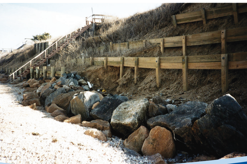
Top photo: This bluff is eroding; the face is unvegetated and slumping. As a result, the houses on top are in danger of sliding off unless immediate action is taken. Bottom photo: This bluff is stabilized by terracing the slope and installing a rock revetment at the toe. Image credit: Jay Tanski
