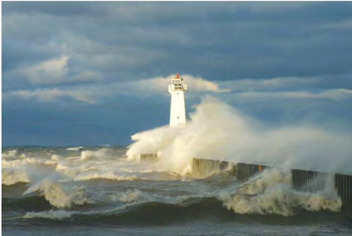
Sodus Point Lighthouse. Crashing waves break over barriers protecting Sodus Point on eastern Lake Ontario.
